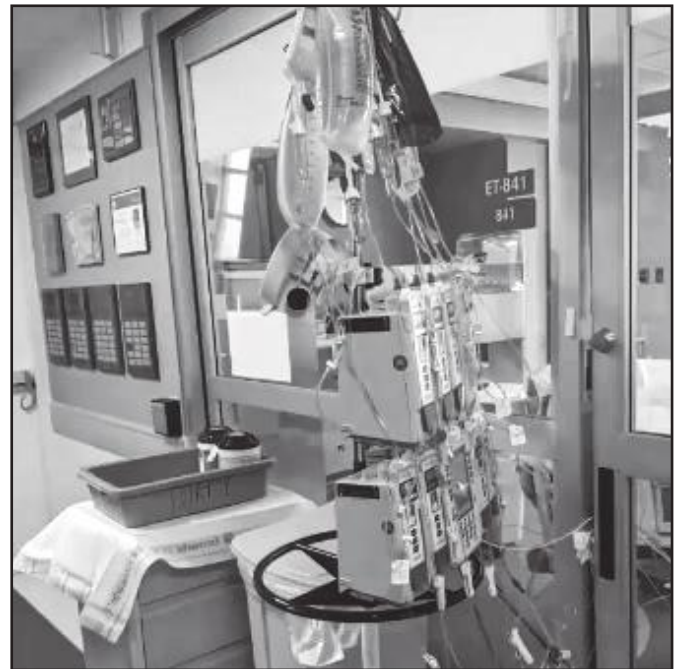
Figure 1. Installation of infusion pumps in the aisle using cord extension to reduce visits of the nursing staff to patient rooms. SOURCE: webcast "Infusion Therapy Conserving Supplies in the Age of COVID-19" ( https://www.ecri.org/landing-covid-infusion-therapy , designed by ECRI and ISMP).
